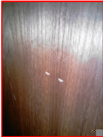
Door to Sitting Room Door Finish - scratched to middle of door panel
