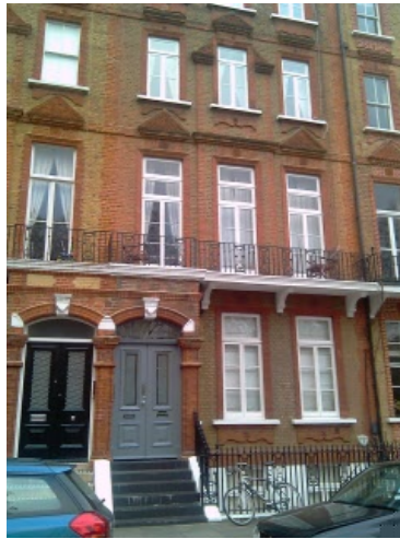
Front of building
