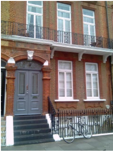
Front of building
