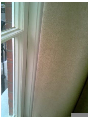
All Windows in Room Full length lined curtains
